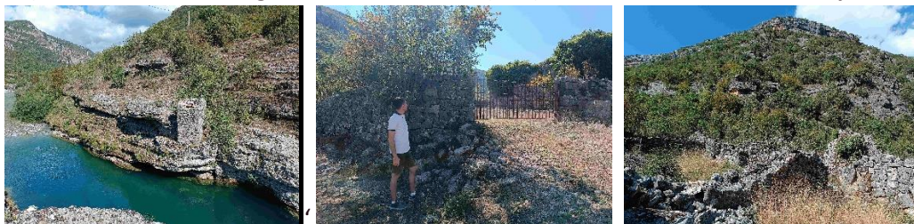
10) Remains of the bridge, watermill and inn ( han ) of Trice in Fu Viza, Cemi - Cijevna Lofka:
